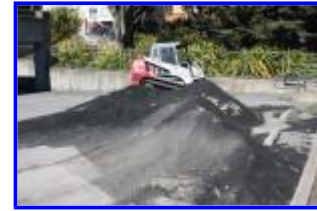
Negoesco Stadium ProTurf Project, 2010 - Mound of rubber pellets removed from old turf.
