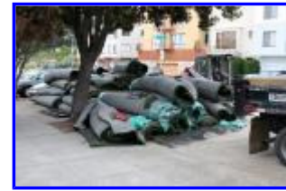
Negoesco Stadium ProTurf Project, 2010 - Old field turf rolled up for removal
