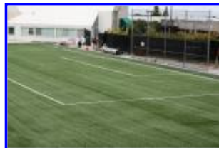
Negoesco Stadium ProTurf Project, 2010 - Turf installed, stitched together and lined
