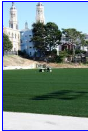
Negoesco Stadium ProTurf Project, 2010 - New turf laid in place, lines complete. Tractor at midfield spreading rubber pellets.
