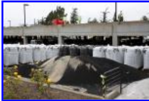
Negoesco Stadium ProTurf Project, 2010 - Mound of rubber pellets removed from old turf in front of bags of new pellets awaiting installation.
