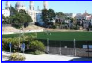
Negoesco Stadium ProTurf Project, 2010 - New turf laid in place and ready to be sewn together.
