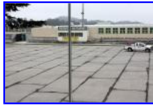
Negoesco Stadium ProTurf Project, 2010 - Old turf completely removed.
