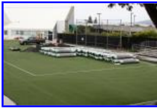
Negoesco Stadium ProTurf Project, 2010 - Old field turf rolled up for removal
