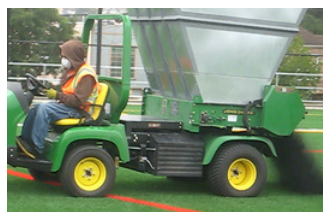
Spreading tire crumb
