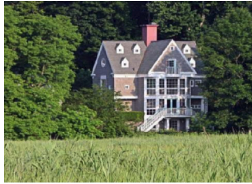
The view of 118 Wilton Road with Taylortown Salt Marsh in the foreground
