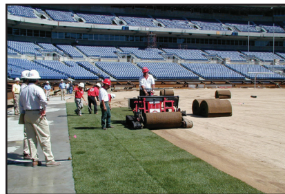
Example of laying sod on a football field. Photo: Ross Kurcab, CSFM
