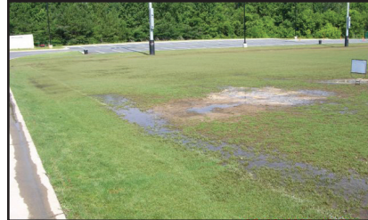
Poor field drainage on a soccer field improperly constructed. Photo: Tony L. Strickland, CSFM
