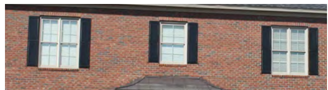
Inappropriately Scaled Shutters.
