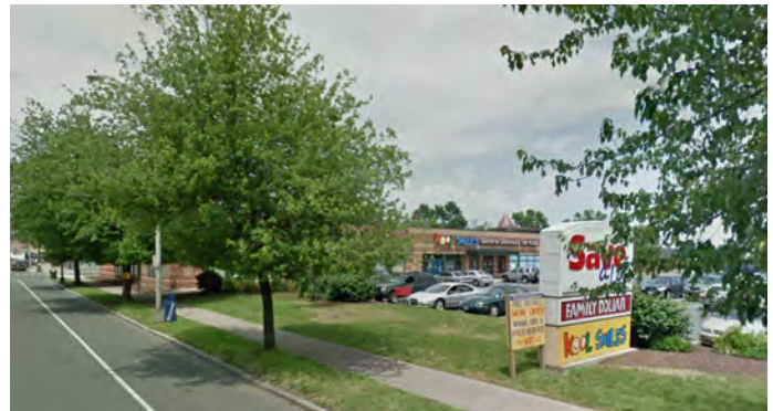
Figure 4.7-A Illustrative Examples of Commercial Center Buildings
