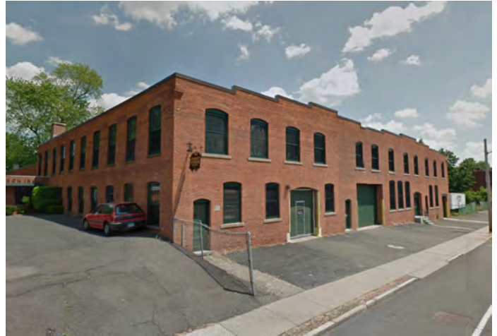
Figure 4.9-A Illustrative Examples of Workshop/Warehouse Buildings
