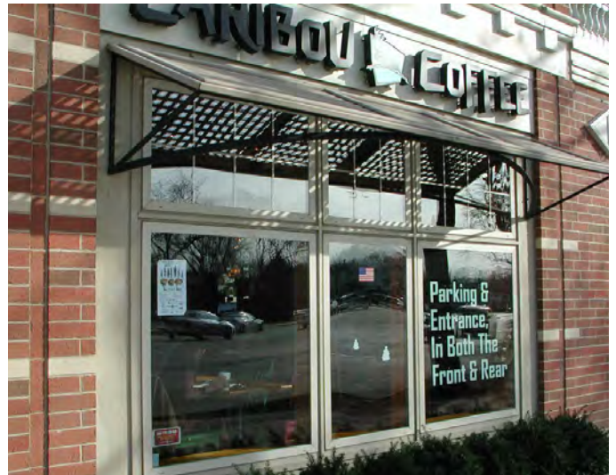
Permitted Awnings: Metal
