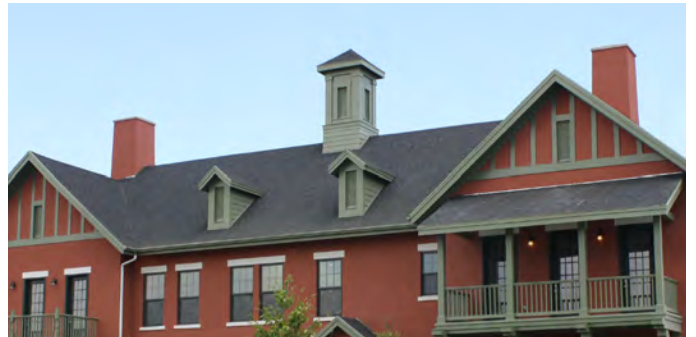
Roof Materials: Asphalt Composite Shingles
