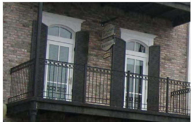
Appropriately Scaled Shutters.
