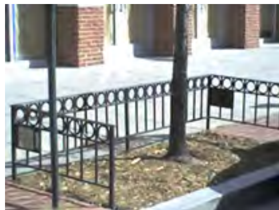
Figure 6.7-A Example of Tree Well Fencing. (photo credit: District Department of Transportation, DC.gov)
