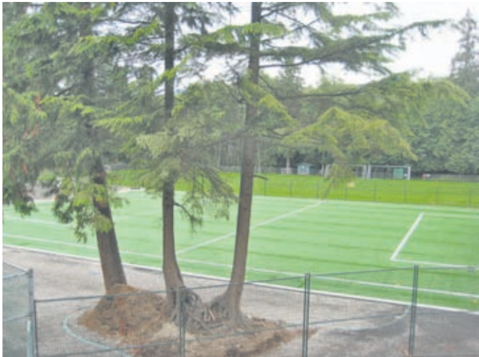
Turf Field ALL LINED UP - the lines are actually permanent white turf and not chalked lines photo by Christine Walker
